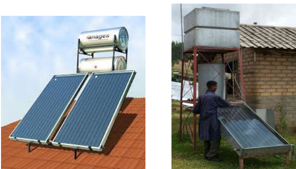
Fig. 5. SWH system with horizontal storage tank (left) and SWH system with vertical storage tank (right)
